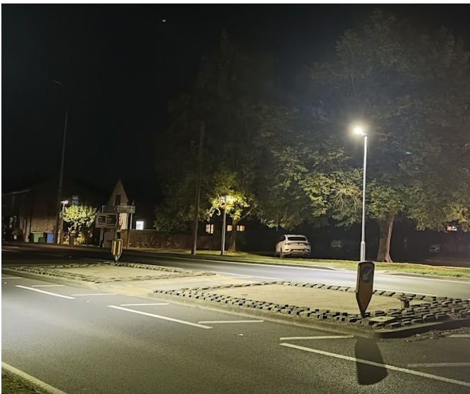
A pedestrian crossing area in Hayton Village remains lit to increase safety for vulnerable road users.
