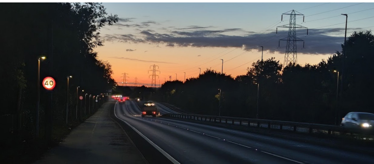
Updated street lighting now features pedestrian-specific lights and solar-powered road studs on a high-capacity dual carriageway.
